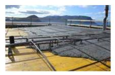
Mix of Dramix® and post-tensioning replace traditional passive reinforcement in on-grade applications
