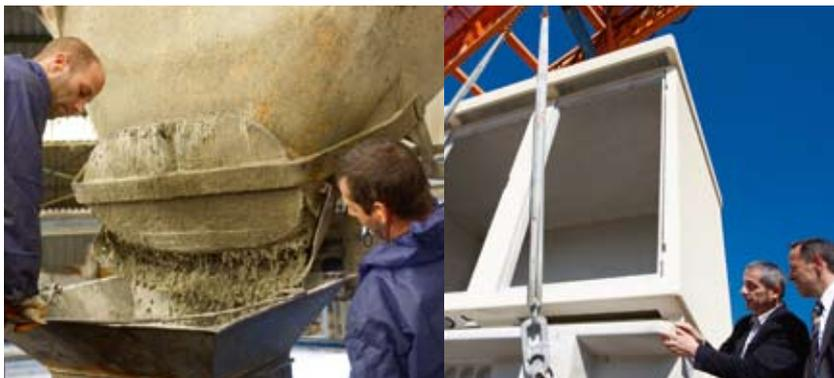
When concrete reinforced with Dramix® Green fibers is discharged, the mix retains its homogeneity
